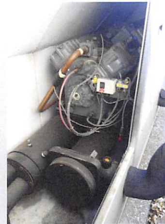
Semi-hermetic compressor with heat exchangers
