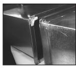
16. On the mating Ductmate frame apply 440 gasket only to the corners as in photo (approximately 3" per corner). The same 3 point application requirements apply as in photo 14.
