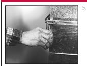
Align duct sections to be connected. Bolt duct sections together at all four corners using 1" x 3%" bolts for the Ductmate 35 system and 1" x <sup>5</sup>/16" bolts for the Ductmate 25 Systems. Do not use the Ductmate "no bolt clips" for removable duct applications.
