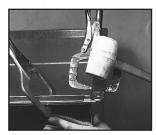
8. Use a mallet to seat the frame onto the duct.
