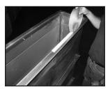
13A. System '45' requires 1" Ductmate 440 Gasket Tape. Start applying halfway between duct corners. Position on inside edge of Ductmate angle as in photo.
