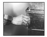
Carefully align mating frames before they touch. Ductmate 440 adheres on contact. A drift pin can be used to correct any misalignment.
