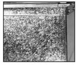
It is essential that the frame angle is fastened to the duct within <sup>3</sup>/<sub>4</sub>" of the end of the angle at each corner.
