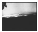
Apply 440 gasket completely around Ductmate frame to the beginning point. Where gasket meets overlay about 3%".
