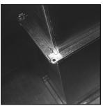
20. Repeat the process at each corner of duct for a quick, strong, good-looking, permanent, no-leak connection of uniform quality every time.
