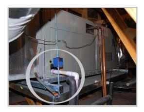
For commercial installations, use threaded rod for added support!
