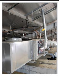
The use of cable & cable locks allow for the bolt to be set in a variety of places with a maximum cable angle of 45°
