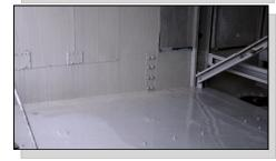
**PANSEAL** is a unique, 100% solids, multi-component epoxy designed to quickly seal and repair leaking and corroded surfaces, forming a new, non-rusting and permanently restored surface. PANSEAL is used worldwide in the HVAC industry to coat, repair and protect cooling towers, chillers and walk in refrigerator rooms.
