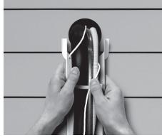
(3) Secure optional SL300 straps (strap kit not included) evenly spaced inside Slimduct. Run lineset, drainhose, wiring etc. over the fitting/duct bases and straps. Tighten straps to secure.
