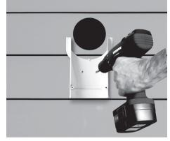
(1) Determine the path which the lineset will follow and strike a chalk line to mark the surface material. Attach the base only of all fittings first (ducting will be placed last), along the marked path, using fasteners of sufficient length (not provided). Predrill where necessary. Duct must terminate with a fitting to prevent cover from sliding out of position.
