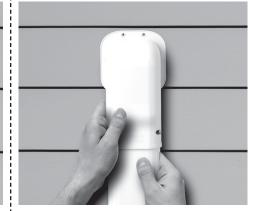
(4) Snap straight duct top over mating straight base pieces. Seat fitting tops over mating fitting bases and secure with provided stainless screws. Duct must terminate with a fitting to prevent cover from sliding out of position.
